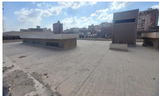
“Case-Study” building Roof
